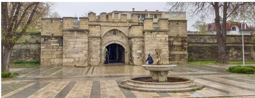
Fig. 44_43 / The refurbishment of Vidin synagogue on the Danube riverfront historic promenade (Author: G. Georgiev)
