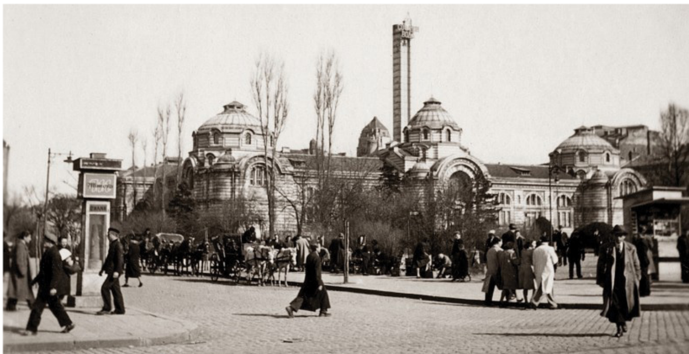
Figure 16. View to the Mineral Bath from the Maria Luiza Blvd. and Ekzarh Yosif St. Junction. Photo www.stara-sofia.com
