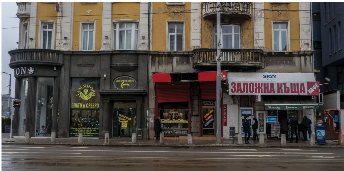
Figure 29. Ground floors that are in bad condition and have not been designed in compliance with the historical facades. Photo Miglena Popova-Vassileva
