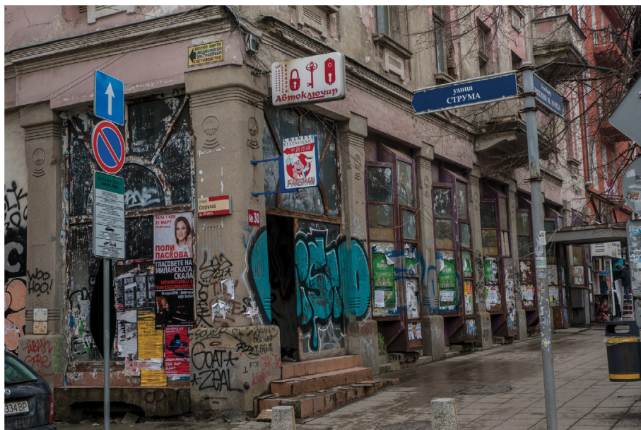
Figure 26. The broken ground floor of the Paris Hotel. Photo Miglena Popova-Vassileva
